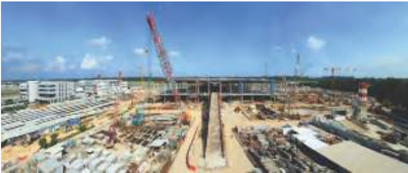
The T4 development project is one of the many projects CAG's Engineering and Development Group manages in entirety from planning and construction to completion.
