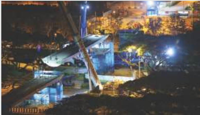
The installation of the final beams on the T4 pedestrian bridge across Airport Boulevard took months of meticulous planning and precise implementation to minimise inconvenience to road users.
