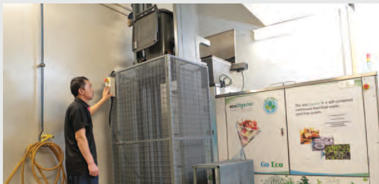
The half-tonne food waste digester handles about 300 kilograms of food waste every day.
